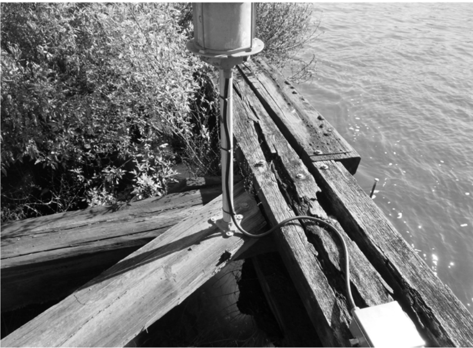
TYP. EXISTING SIGNS AND CONDUITS TO BE REMOVED AND REINSTALLED AS NEEDED
