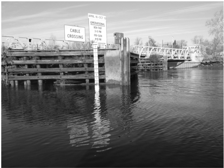
TYP. EXISTING CLEARANCE GAUGE
