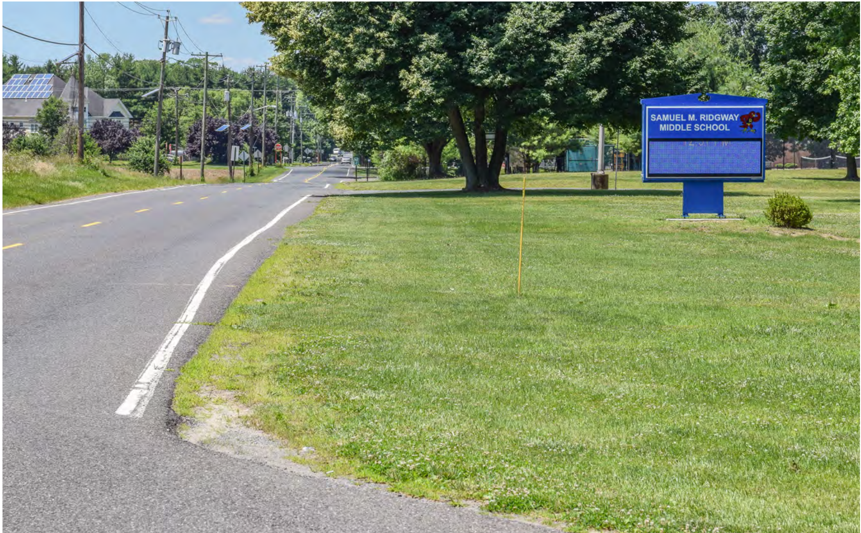
Delanco Road lacks pedestrian facilities near the Township Middle School
