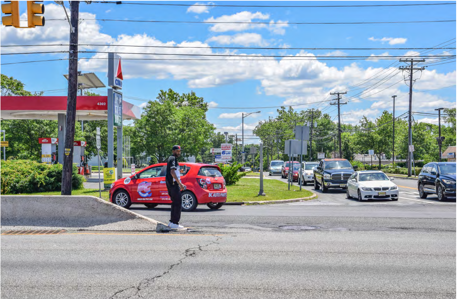
The intersection lacks pedestrian facilities, forcing pedestrians to cross unsafely
