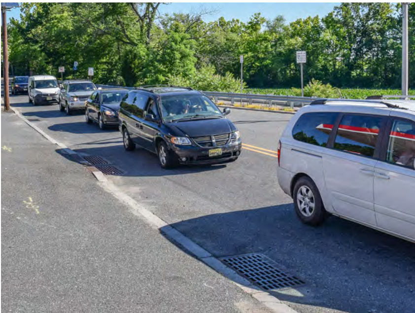
Off-peak queuing regularly occurs at the intersection due to a lack of dedicated turn lanes
