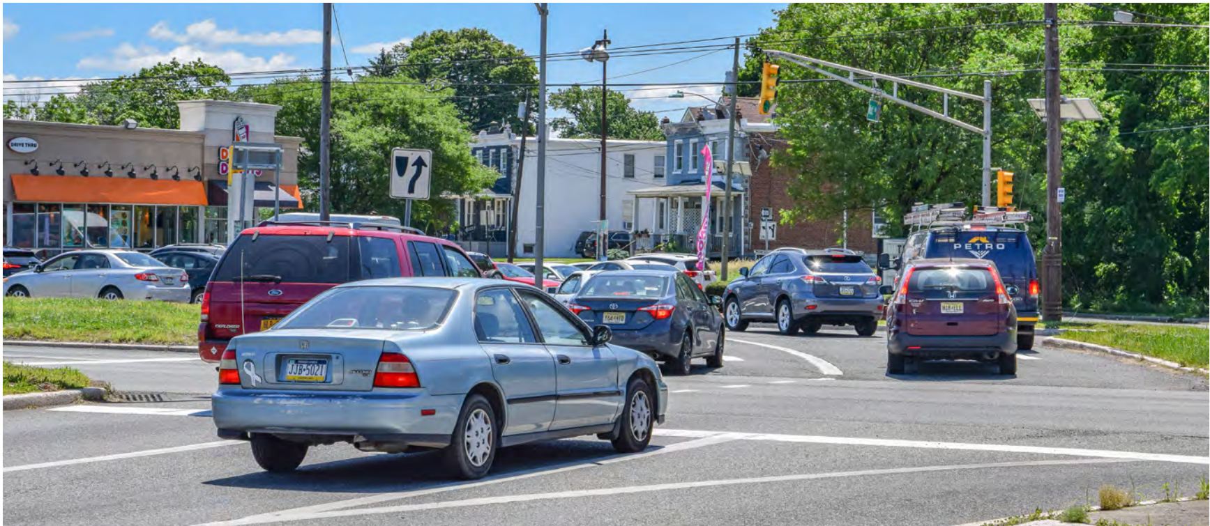
During the green phase, left-turning vehicles from NJ 413 to northbound U.S. 130 have little room for stacking due to the simultaneous red light at the Lincoln Avenue signal just 500 feet to the north
