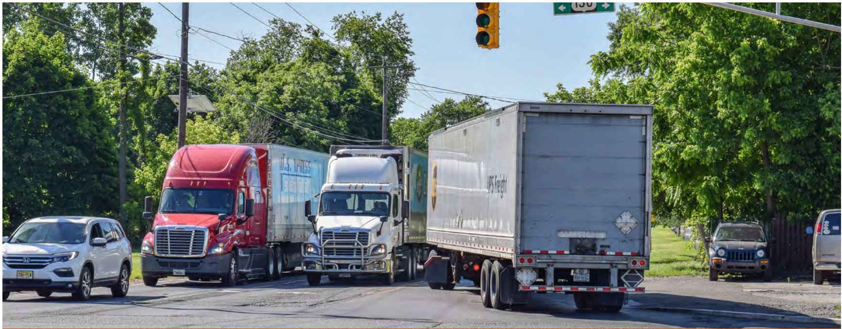
Lack of a channelized right-turn lane from northbound U.S. 130 to Florence-Columbus Road results in truck congestion at the intersection
