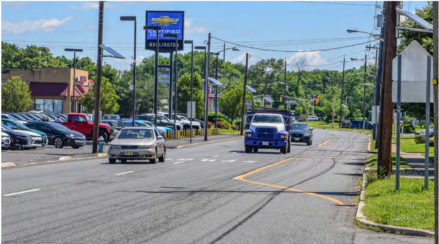
Recently implemented road diet along southbound U.S. 130 approaching High Street (CR 541)
