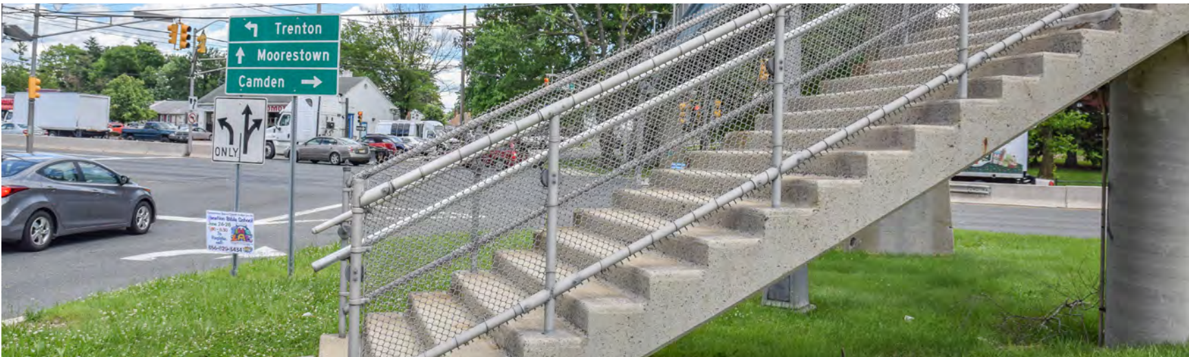
The existing pedestrian bridge over U.S. 130 is obsolete by current ADA requirements
