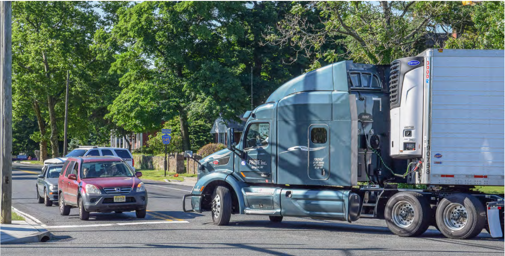
Right-turning trucks from northbound U.S. 130 to eastbound Farnsworth Avenue have limited space due to a tight curb radius
