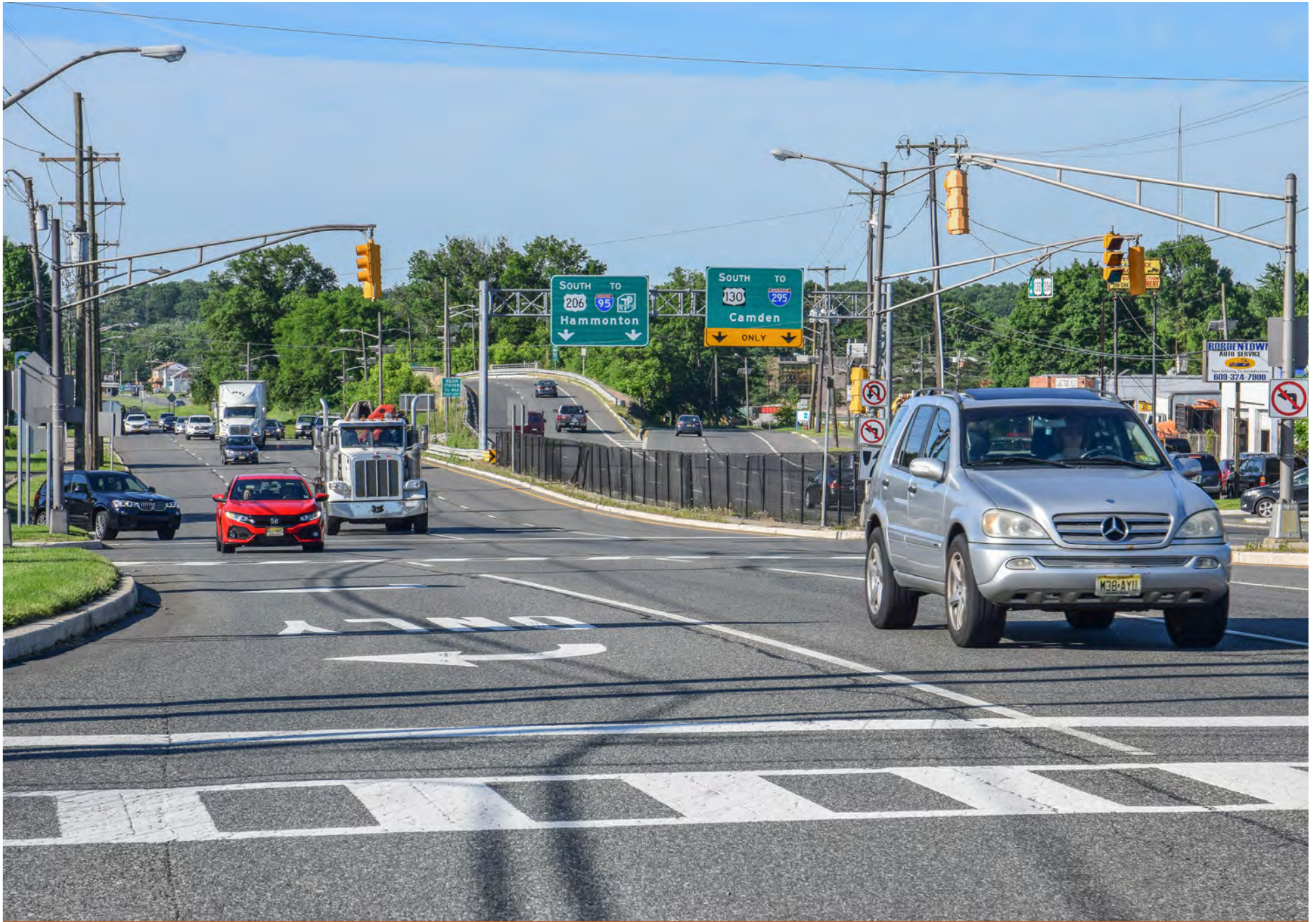
U.S. 130/206 concurrency currently consists of 3-4 lanes in each direction with minimal pedestrian accommodations
