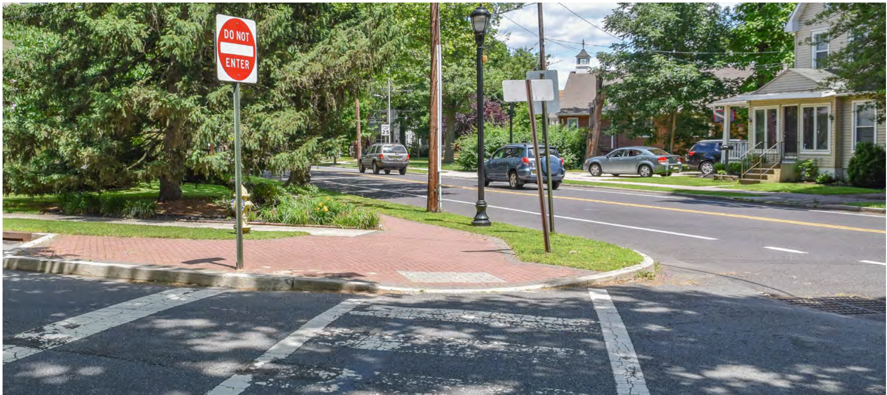
Poor visibility from Willow Street to Burlington Avenue (CR 543)
