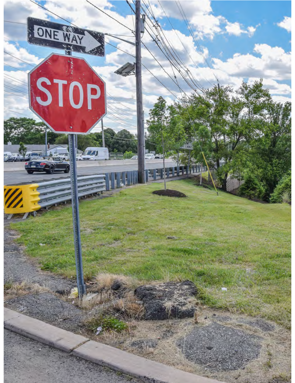
Lack of pedestrian facilities to the south of the intersection
