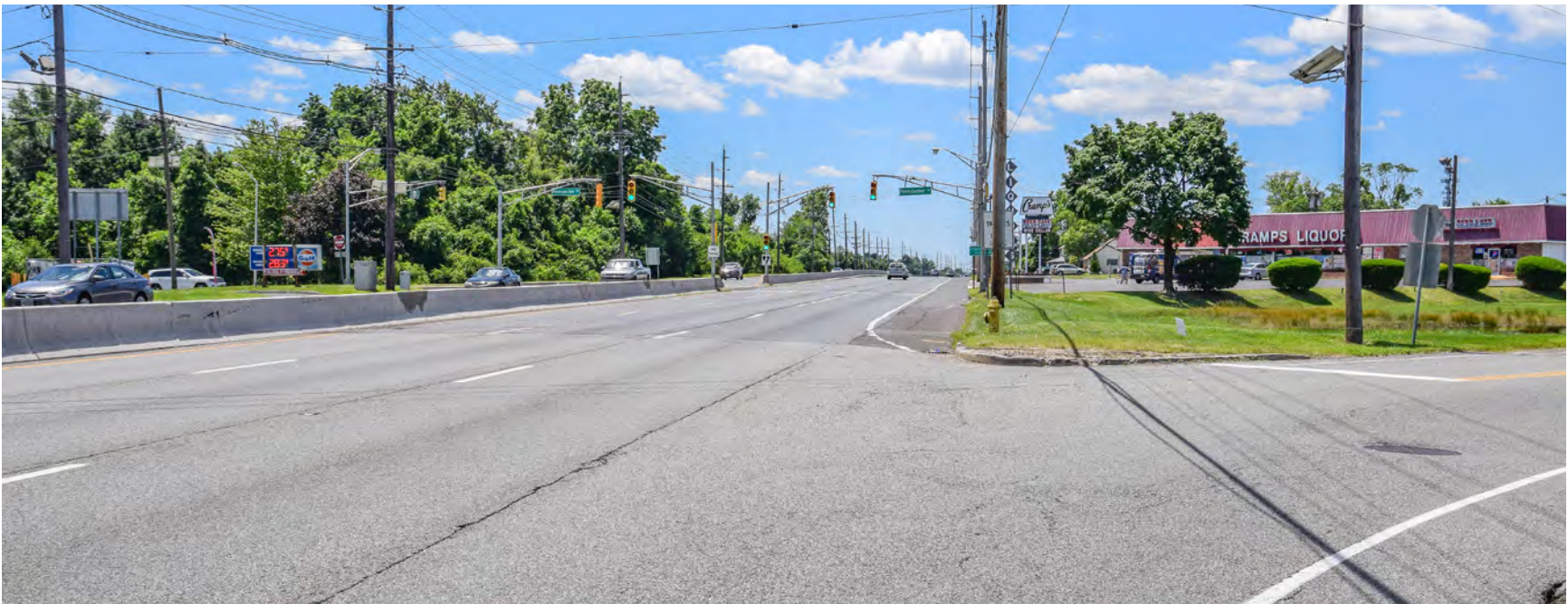
Existing turn to Delanco Road (foreground) with the Pennypacker Drive intersection to the south. The proposed extension crosses the liquor store parking lot to the right and continues to Delanco Road further west
