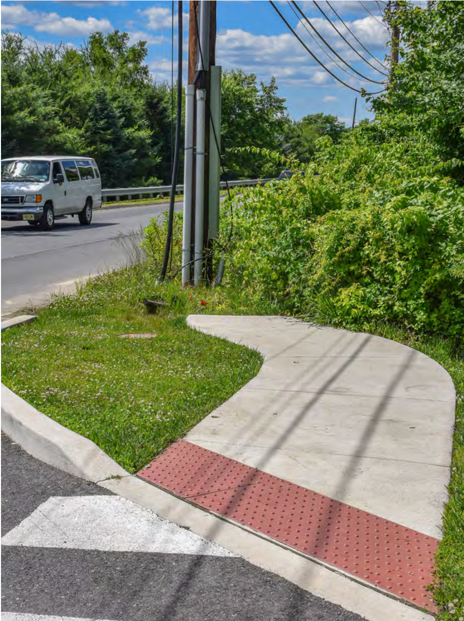
Sidewalk terminates abruptly just north of the intersection
