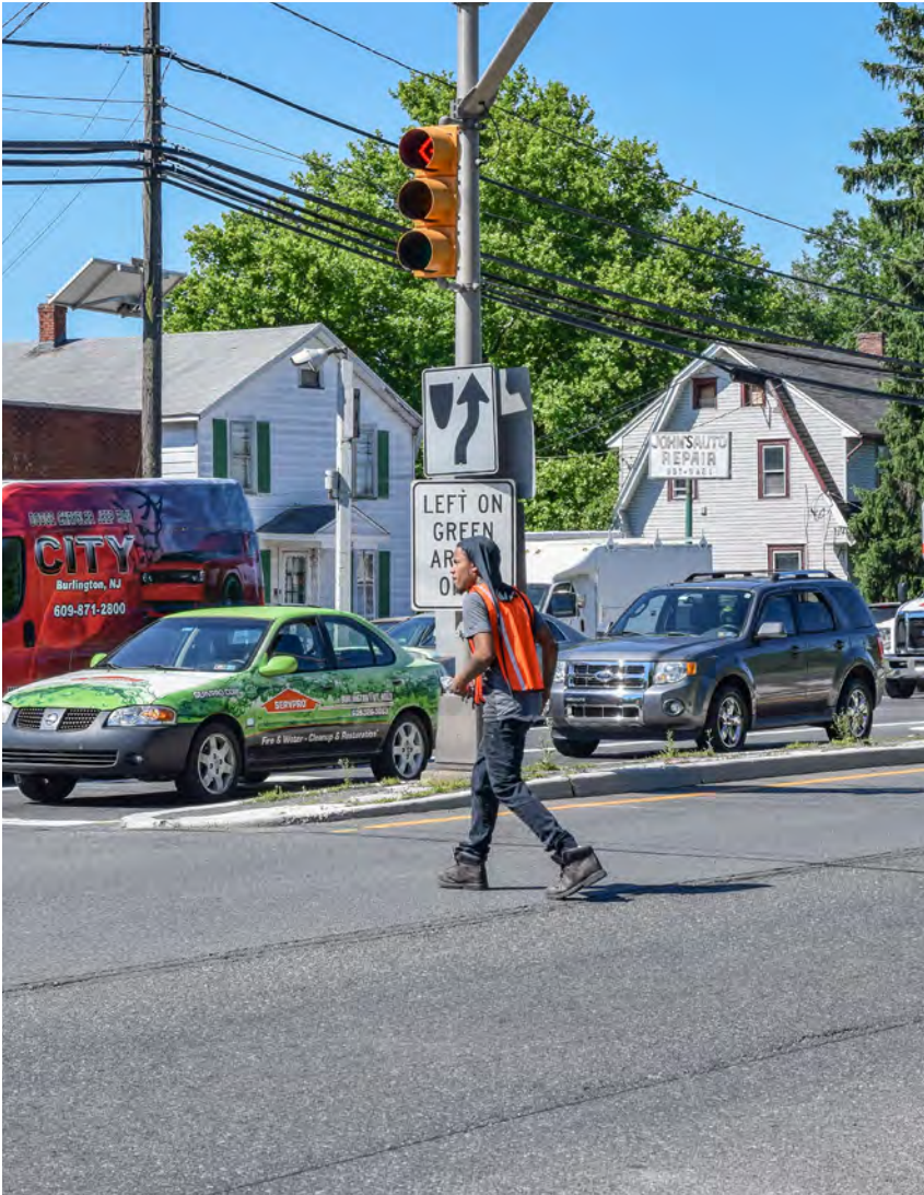
The intersection lacks pedestrian facilities, forcing pedestrians to cross under dangerous circumstances
