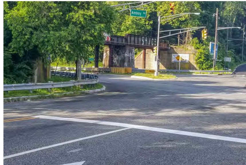
Insufficient clearance for right-turning vehicles from northbound U.S. 206 to Amboy Road
