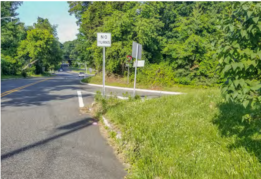
Poor visibility of the jug-handle merge for westbound traffic on Amboy Road due to excess vegetation
