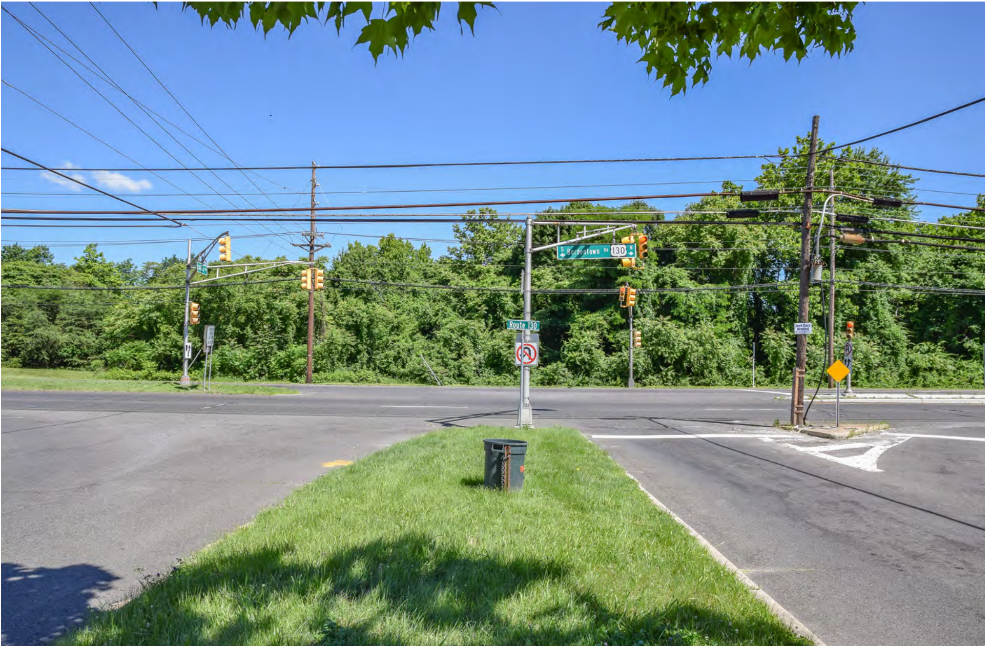
The existing northern terminus of La Gorce Boulevard at U.S. 130
