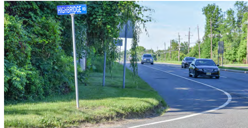
Limited visibility, lack of deceleration lanes, and poor advance signage at the intersection
