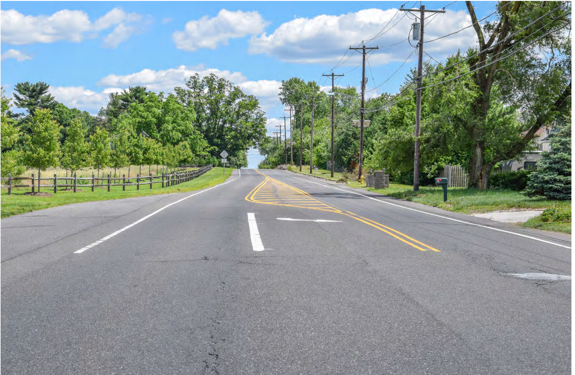
Traffic calming may be necessary near the Laurel Run Park driveway to reduce vehicular speeds and provide for adequate pedestrian crossings
